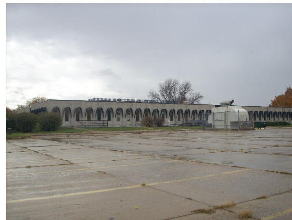
4. View of Iowa Telecom site facing southwest
