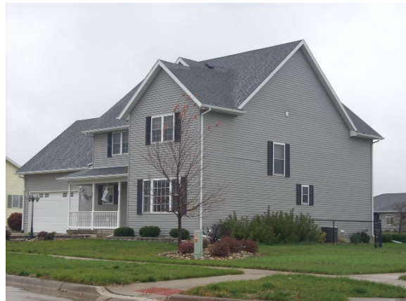
9. View of an existing home in East Gate
